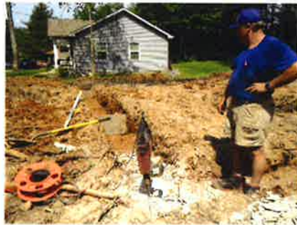
James Hembre works on digging the Footers
